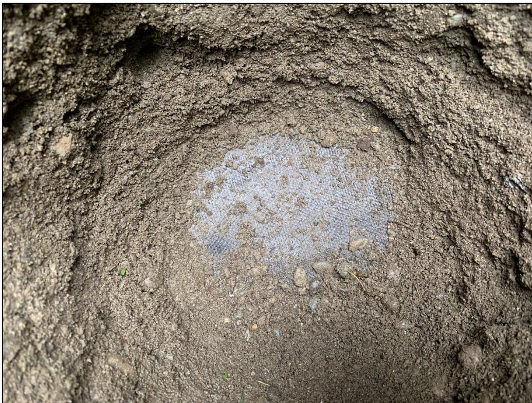
Figure 27: Filter fabric at bottom of ST 7.
