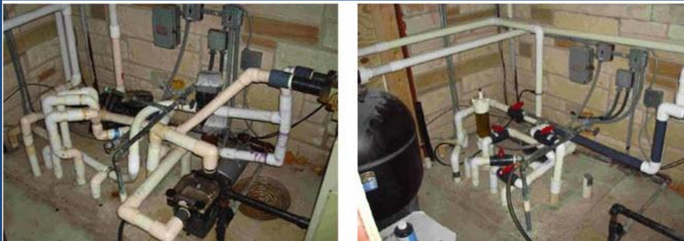
Effects of low alkalinity on left (plumbing corrosion)
