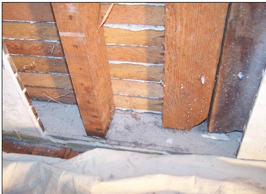
Figure 4. Interior wall cavity, Smith House, 2006.
