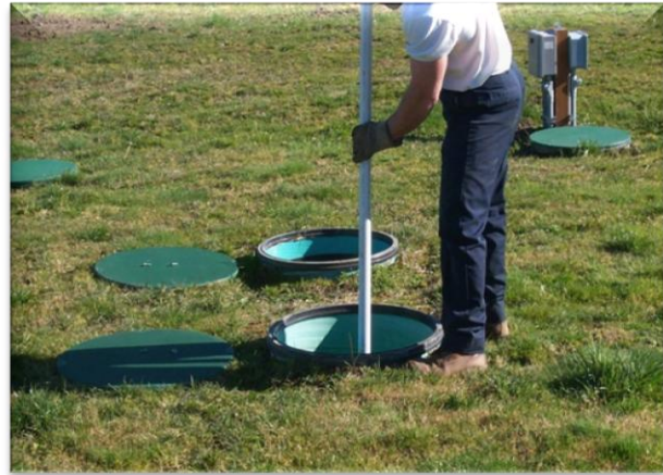
Septic tank inspection in process
