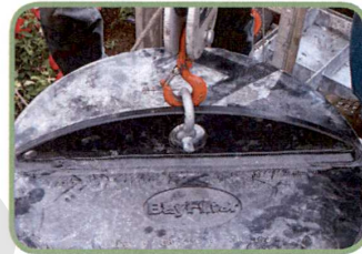
Cartridge Hoist Point
