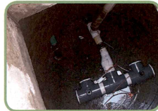
Manifold Tee View of a Cleaned System
