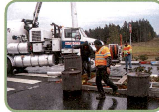
BayFilter System Cleanout
