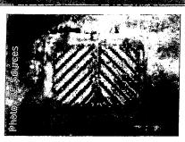
You will often see fabric filters placed in these catch basins near construction sites. These filters are designed to keep out large debris but do not capture silt or other fine material. They should be changed whenever they are torn and monitored in case they become clogged. Filters should be removed after construction is complete.
