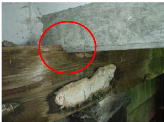
Crushing of the pier cap
