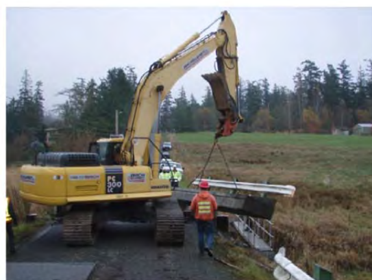
Removal of bridge girders
