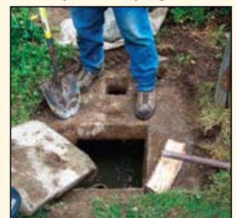
Septic tank baffle screen inspection in progress
