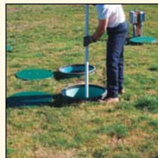
Septic tank inspection in progress
