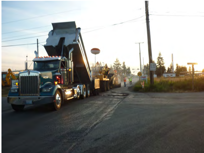
Asphalt Overlay Program in 2013
